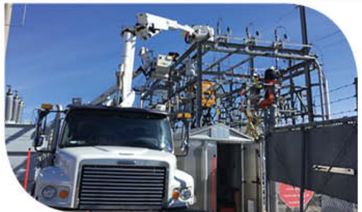
▶ Another LCP line crew doing upgrades to the Cohasset Substation in June. The existing substation regulators are at capacity and were upgraded along with new regulator bypass switches. The high-side fuses will also be replaced with a transrupter. The work will improve reliability for members served by this substation.
